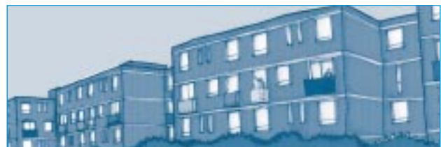
'Fish' balconies after
